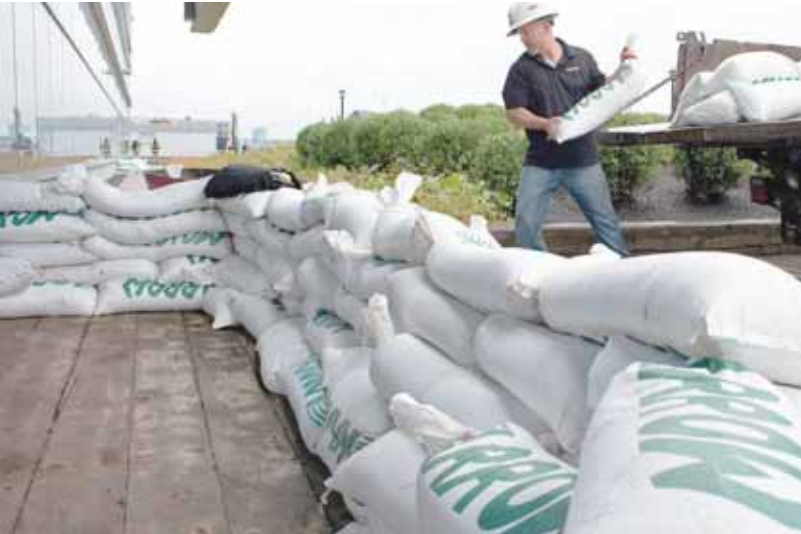
A project manager for general contractor G&R Kelly, places sandbags around the doors of the Nova Scotia Power building before the arrival of Hurricane Fiona in Halifax, Nova Scotia. – Reuters
