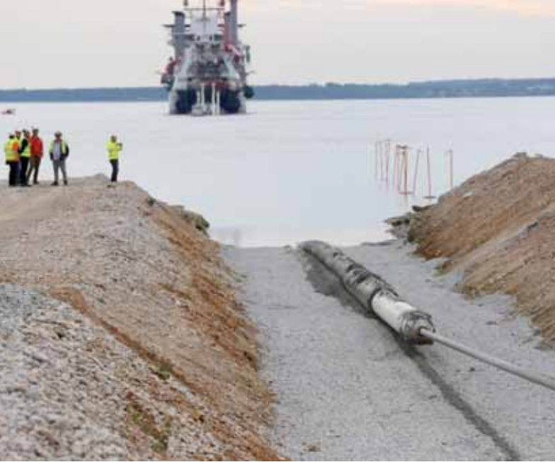
A view of the Balticconnector pipeline as it is pulled into the sea in Paldiski. — Reuters
