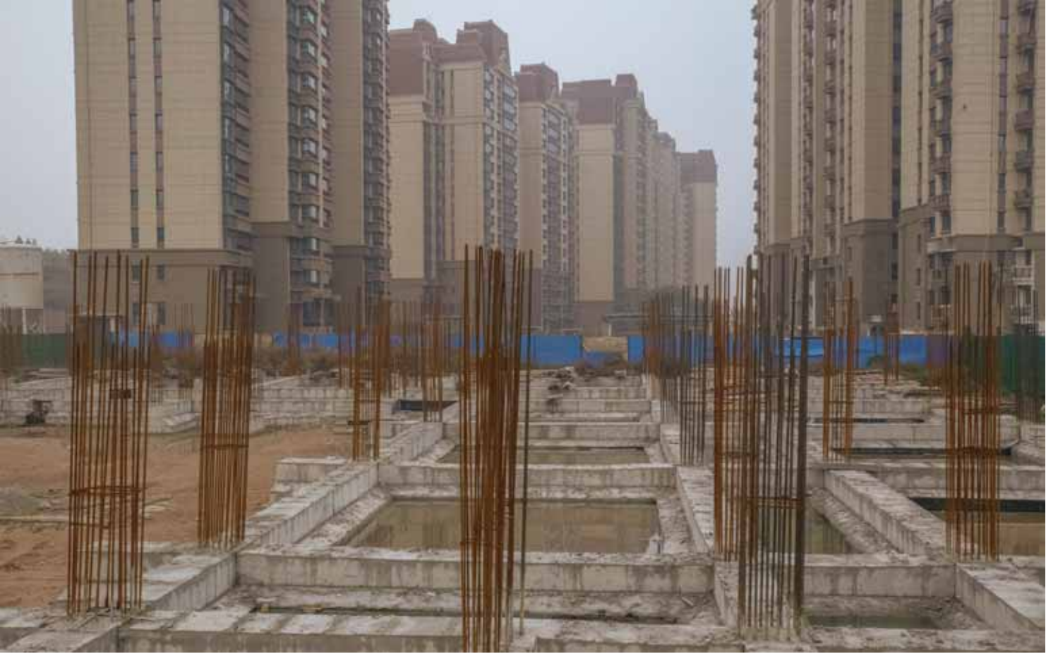
An idle construction site for an Evergrande residential project in Taiyuan, China. – The New York Times
