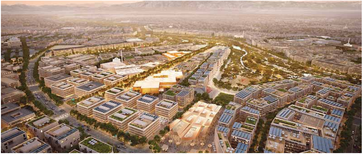
The construction works of the Sultan Haitham City project Phase One have begun.
