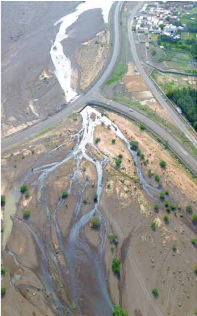
Dams in Mahadha retain 3.3 million cubic metres of water following recent rains.
