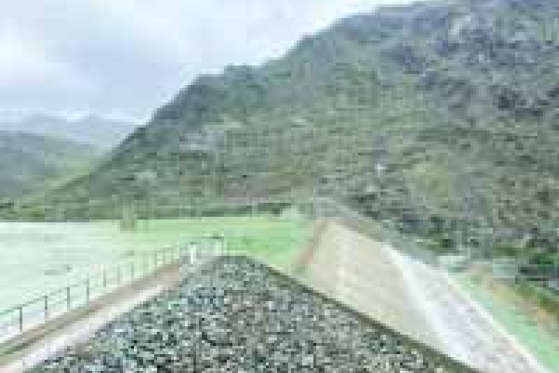
Heavy rains from April 14 to 17 filled or partially filled 49 dams in several governorates.
