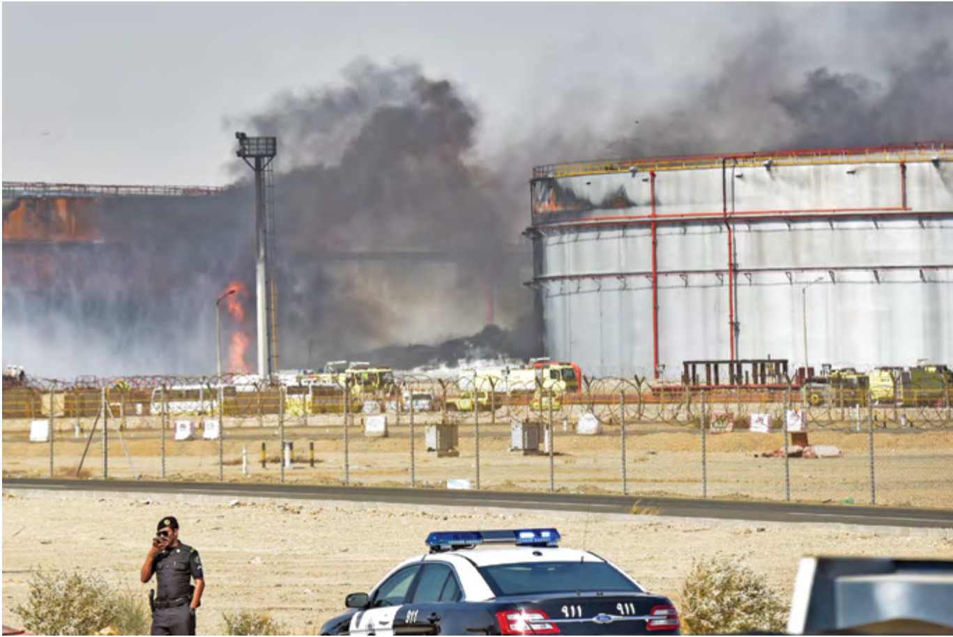
A policeman stands guard as firefighters extinguish fire at a Saudi Aramco oil facility in Jeddah, on Saturday, a day after a Yemeni rebels attack (AFP)
