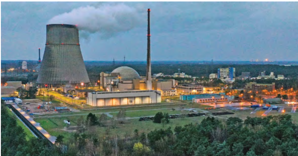
An aerial view of the nuclear power plant Emsland in Lingen, western Germany (AFP)
