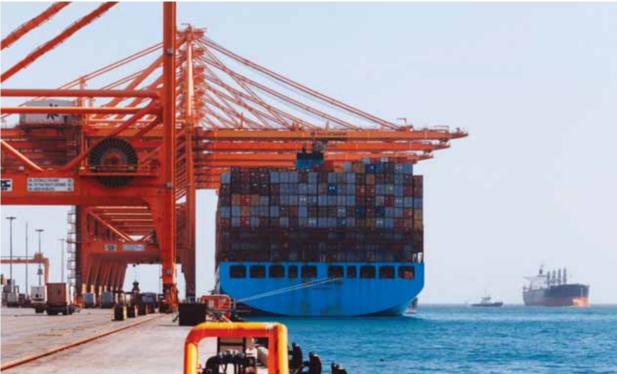
Upgrades to the four berths to support the new cranes have been completed, with two additional berths under construction.
