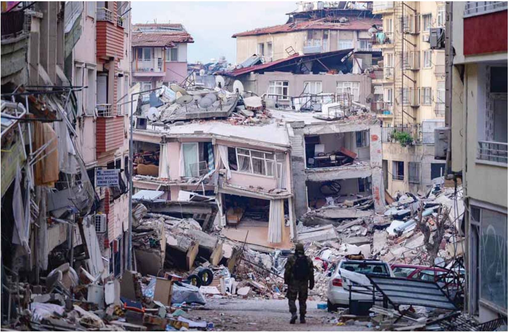
A Turkish soldier walks among destroyed buildings in Hatay after a 7.8-magnitude earthquake struck the country's south-east. – AFP
