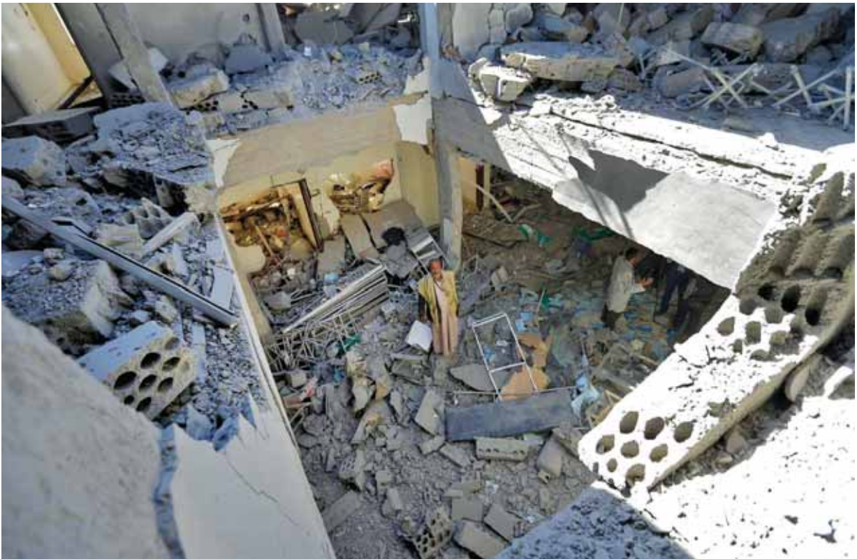
An airport worker walks through the debris of a building destroyed following a reported air strike by the coalition targeting the Ansar Allah-held Sanaa International Airport on Tuesday. — AFP
