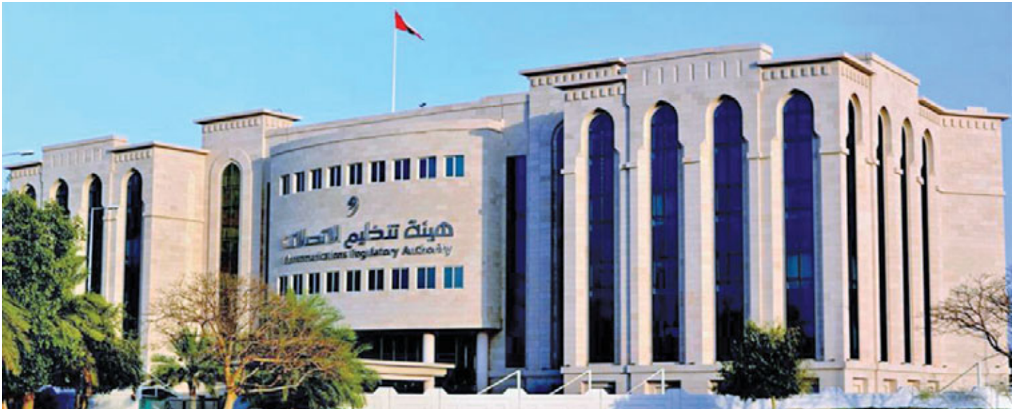
SERVICES: The services include receiving, clearing, sorting and distributing courier, as well as all types of postal letters, including documents, parcels, packs and packages weighing not more than 25 kilograms. - ONA
