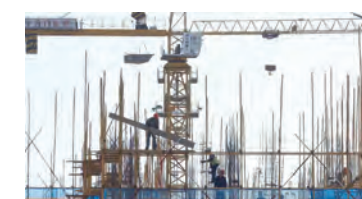
Staff work on a construction site in Dalian, China. — Reuters
