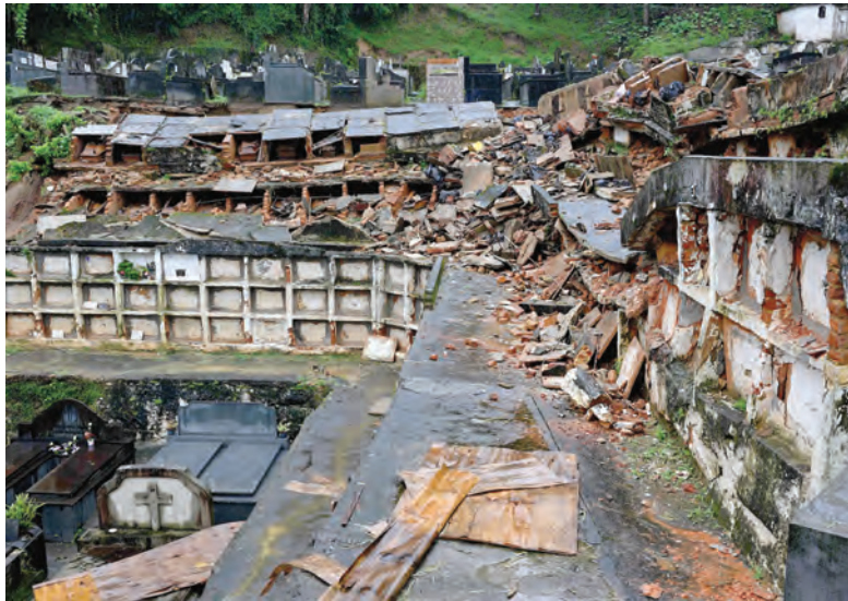
Partial view of the municipal cemetery of Petropolis, where several niches were damaged when they collapsed due to the heavy rains in Petropolis, Brazil. – AFP
