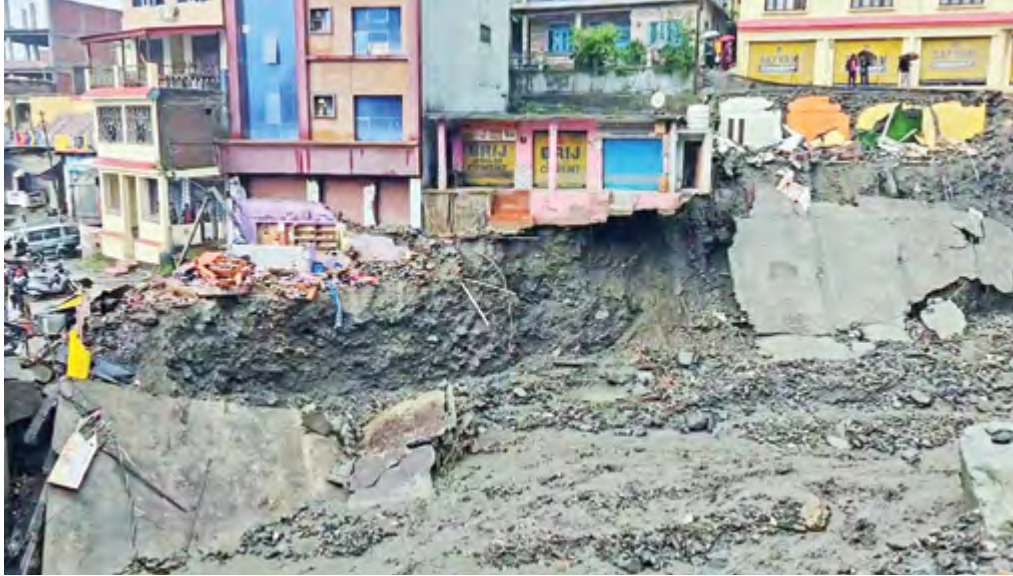
A view of damaged structures and collapsed terrain following a landslide, in Ramban, India on Sunday (ANI)
