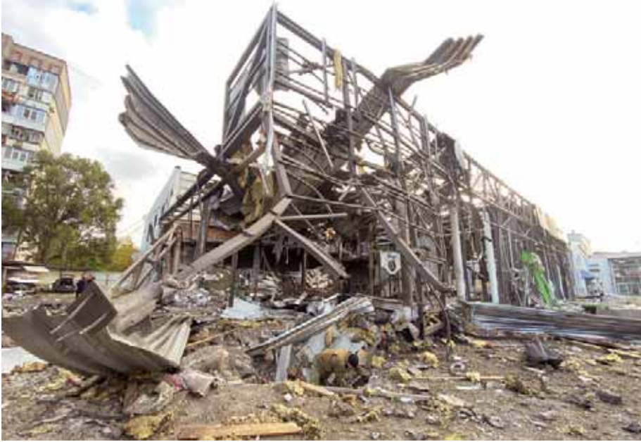
A view shows an office building of a car retailer destroyed during a Russian missile attack in Zaporizhzhia. — Reuters
