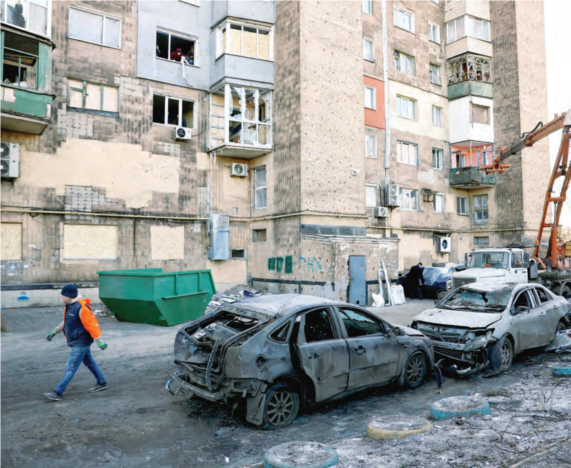
People carry out repair works in the courtyard of a damaged multi-storey residential building following recent shelling, in Makiivka, a Russian controlled region of Ukraine. — Reuters
