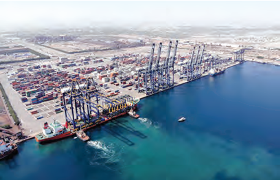
SOHAR Port recorded an exceptional 1,766 % surge in ship destination change requests.
