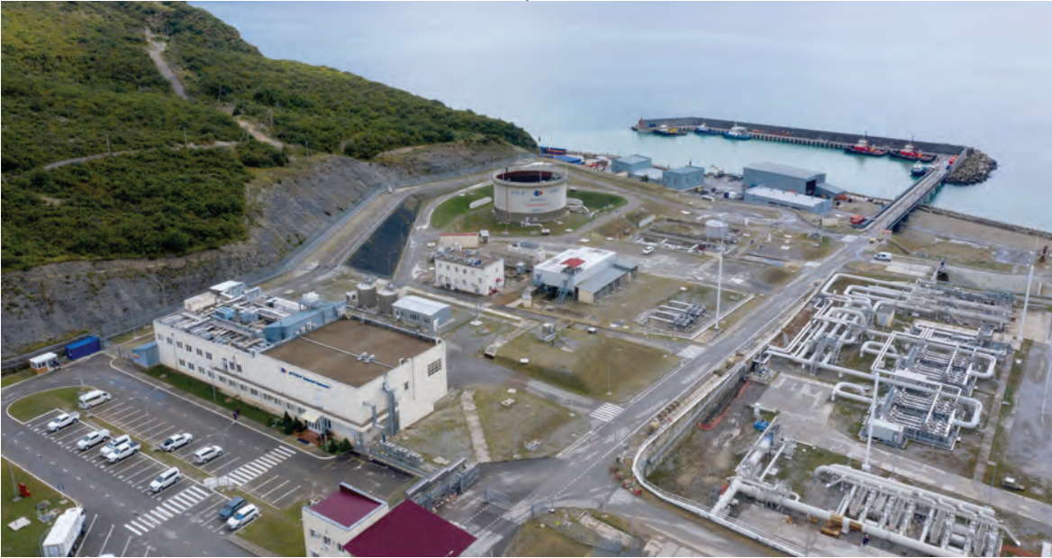
Facilities of the Caspian Pipeline Consortium’s (CPC) Marine Terminal in Yuzhnaya Ozereyevka near the Black Sea port of Novorossiysk, Russia. — Reuters file photo
