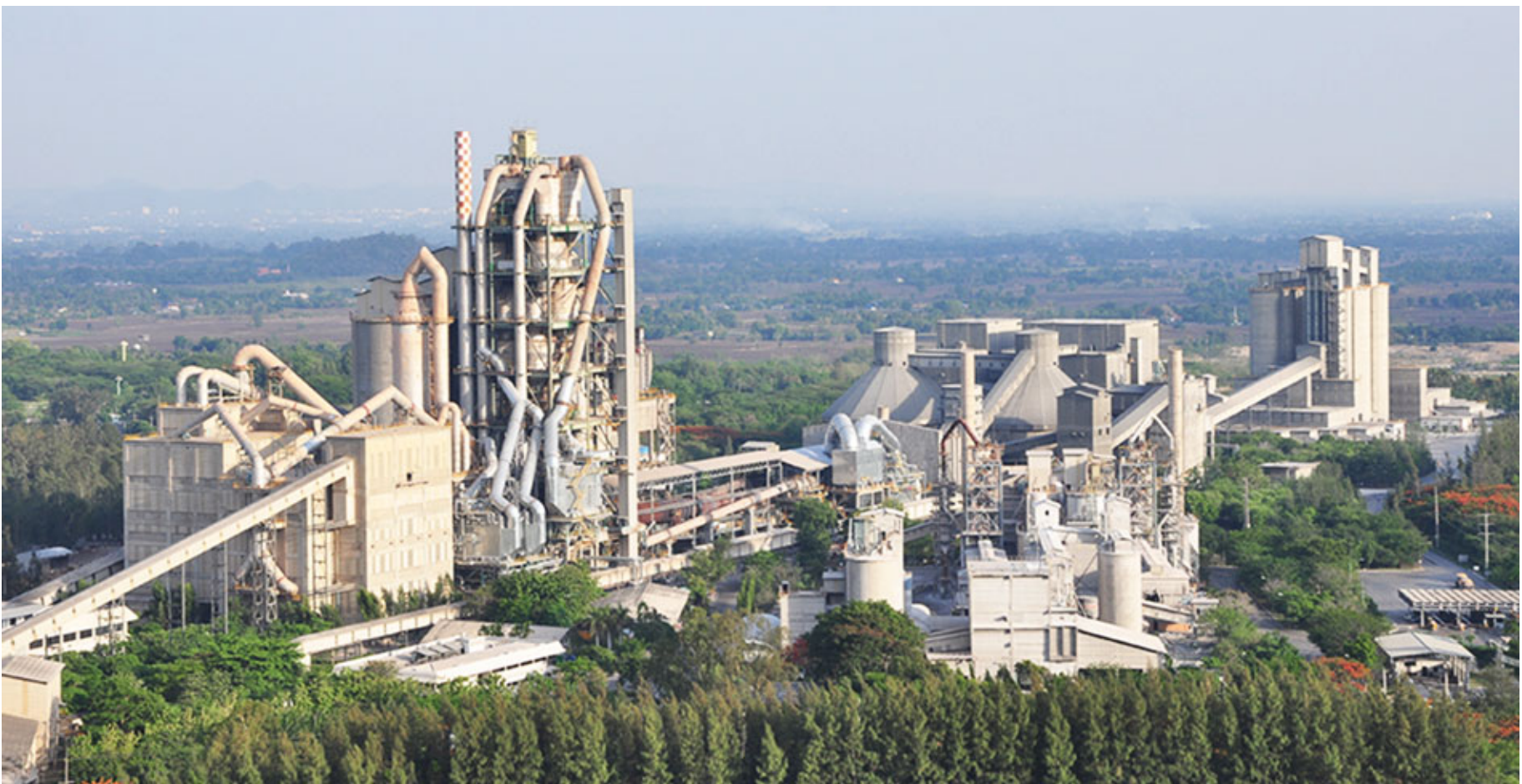
MEETING LOCAL DEMAND: This new plant will help to meet the local demand and the demand in the overseas markets of India, Sri Lanka and East Africa with the support of well-equipped and dedicated port facility at the Port of Duqm. - Supplied picture
