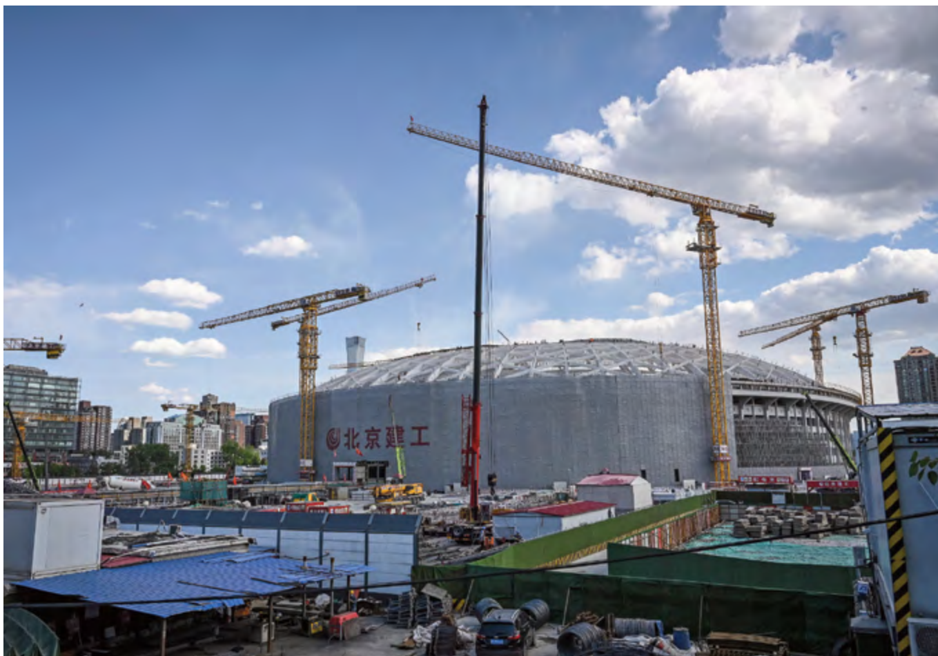
The construction site of the Workers' Stadium, a planned venue of the 2023 Asian Cup, in Beijing on Saturday (AFP)
