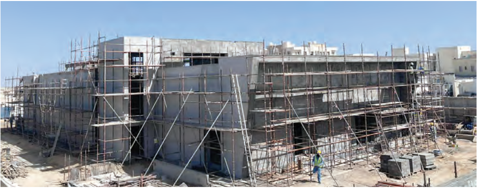
The Advanced Emergency Unit project at Al Duqm Hospital will be opened soon.
