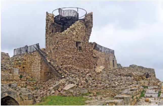
Aleppo's ancient citadel is seen damaged following the deadly earthquake that shook Syria on Monday (AFP)
