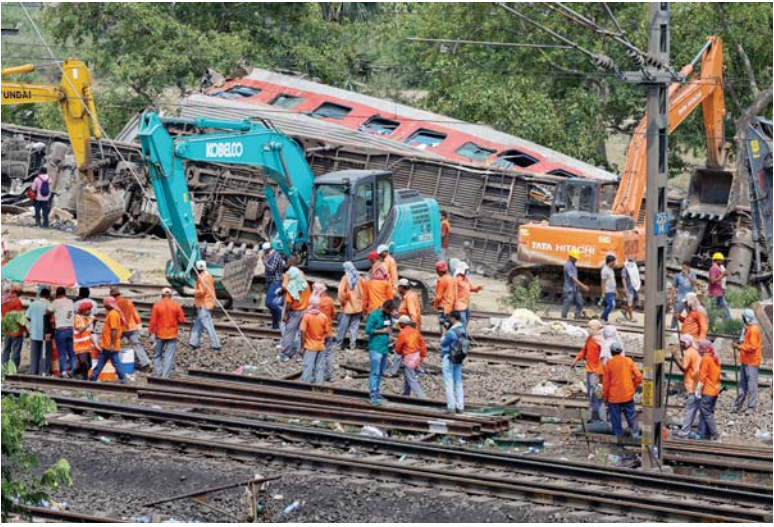
Heavy machinery remove damaged coaches from the railway tracks at the site of a train collision following the accident in Balasore. — Reuters
