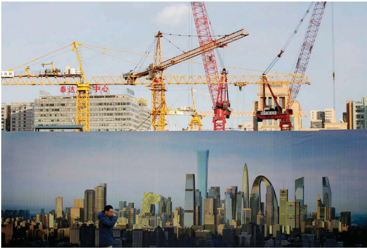
A construction site is seen behind an image of an imagined new skyline, in Beijing. — Reuters
