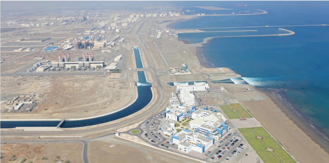
AI-enabled technologies can support the transition of industrial zones to low-carbon clusters.
