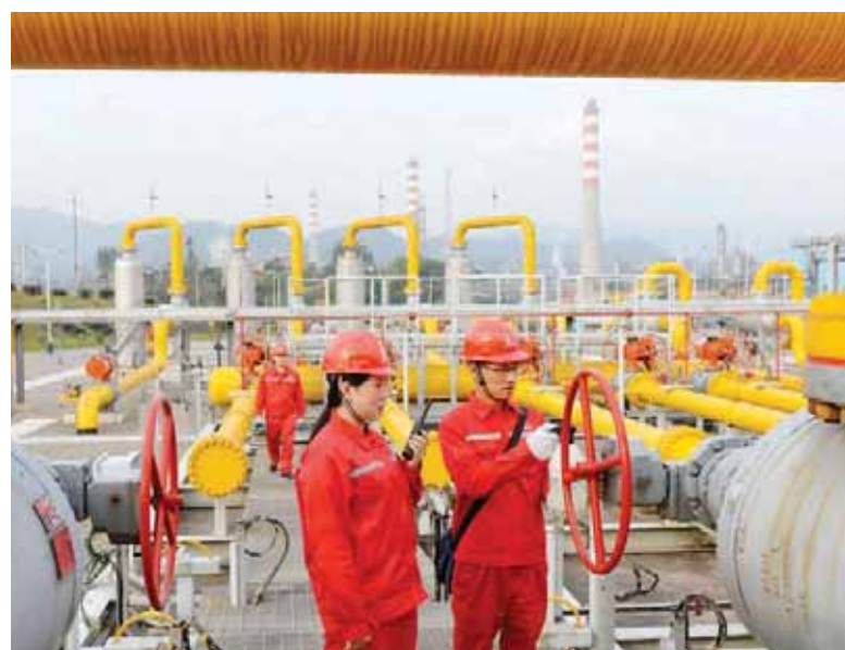
Workers inspect a pipeline at a natural gas facility run by Sinopec in southwest China's Sichuan province. — Reuters
