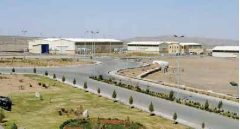
View of the Natanz uranium enrichment facility 250 km south of Tehran. — Reuters
