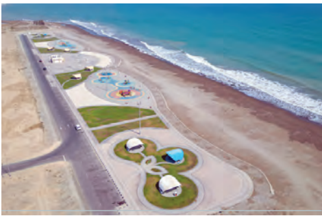
The redevelopment features 989 metres of pedestrian walkways to encourage active lifestyles.
