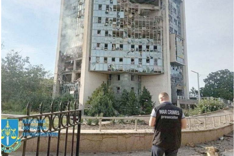
An inspector surveys the damage at a grain port facility after a reported attack by Russian military drones in Izmil on Wednesday. – Reuters
