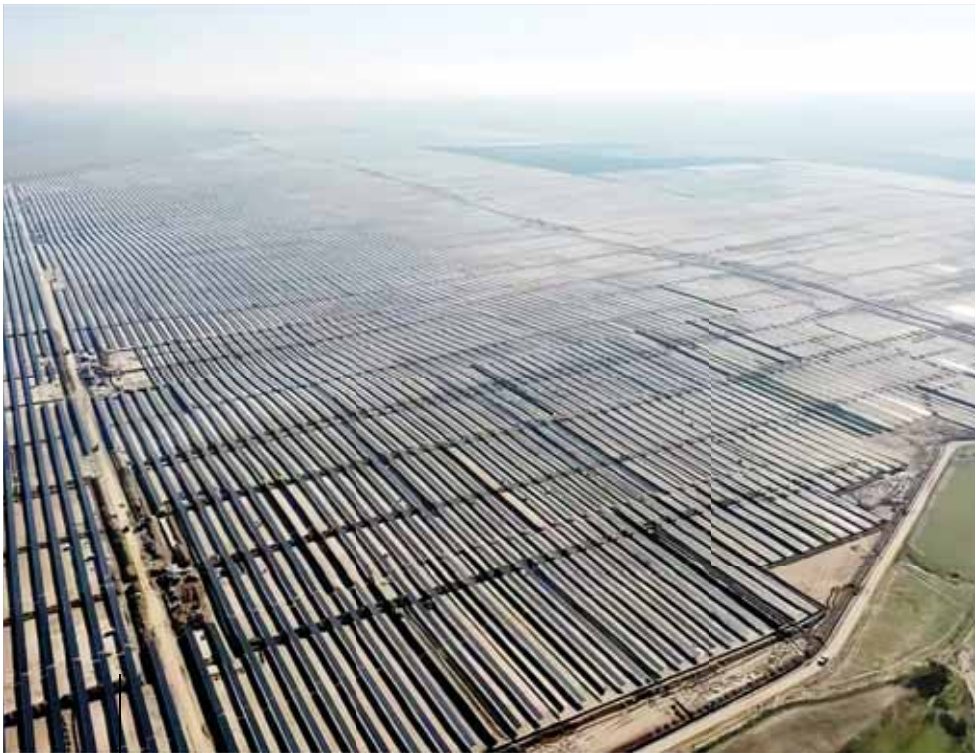
Solar PV plant in Samarkand, Uzbekistan This picture shows the solar PV plant built by China's Dongfang Electric Corporation in Samarkand, Uzbekistan. Xinhua
