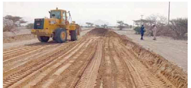
Internal road paving project in the Wilayat of Bidiya is part of a number of projects implemented by the governorate. -- ONA
