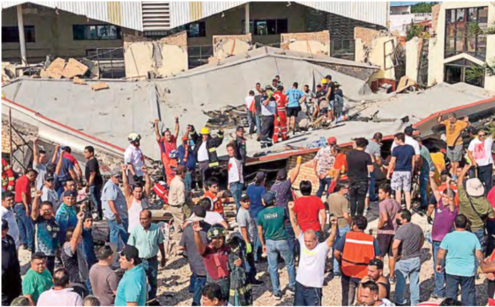
Rescuers working after a church roof collapsed in Ciudad Madero, Tamaulipas State, Mexico, on Sunday (AFP)
