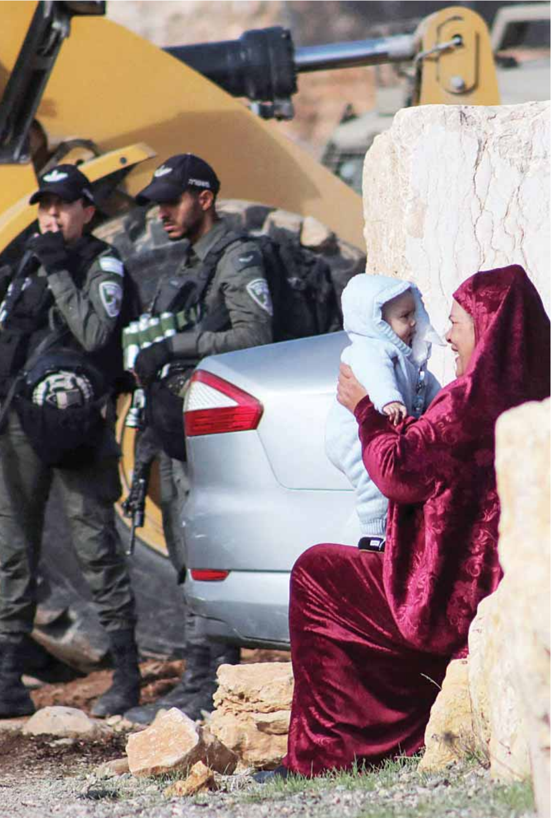
A woman cuddles a baby as excavators of the Israeli army demolish two Palestinian houses in the Jabal Johar area of Hebron city, near the Kiryat Arba Israeli settlement, in the occupied West Bank, on Monday. – AFP
