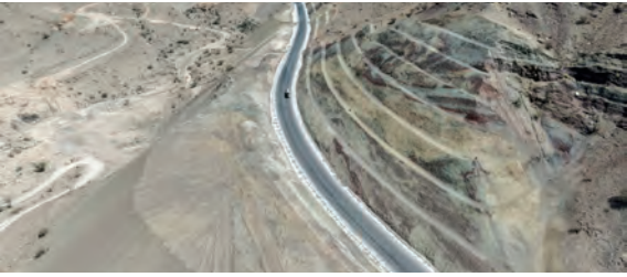
The project costs exceed RO 13 million and spans 9 kilometres.
