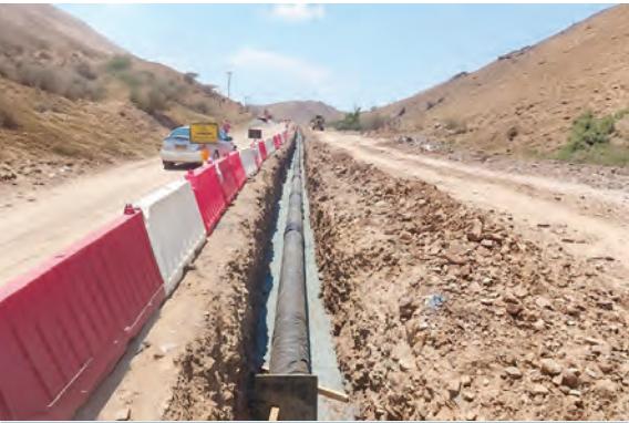
The project included implementation of a water network using HDPE pipes.
