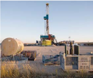
A drilling rig in the early stages of installation near Douglas, Wyo.
