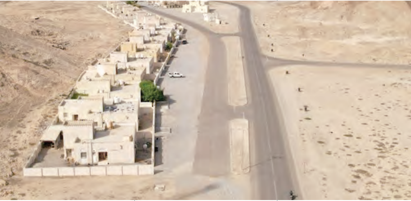
The project has been transferred to Dhofar Municipality and retendered, with the new phase focused on completing what remains of the existing development (Picture for illustration).
