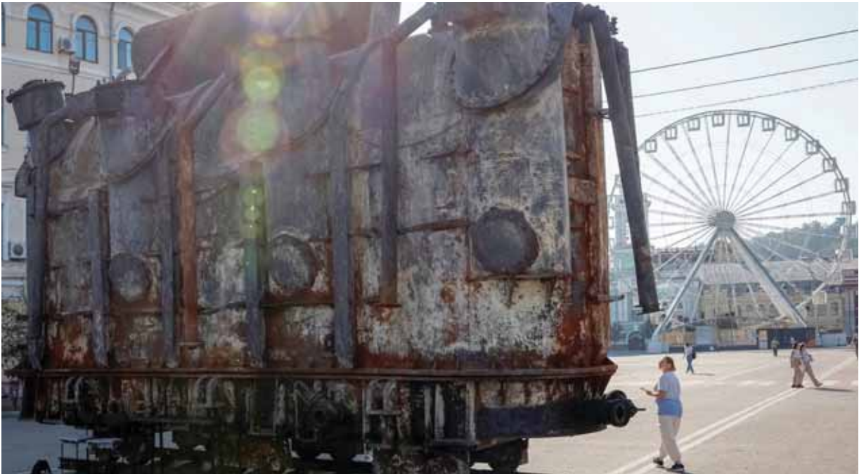
A woman looks at an installation with a power transformer, damaged by a Russian military strike, in Kyiv. — Reuters
