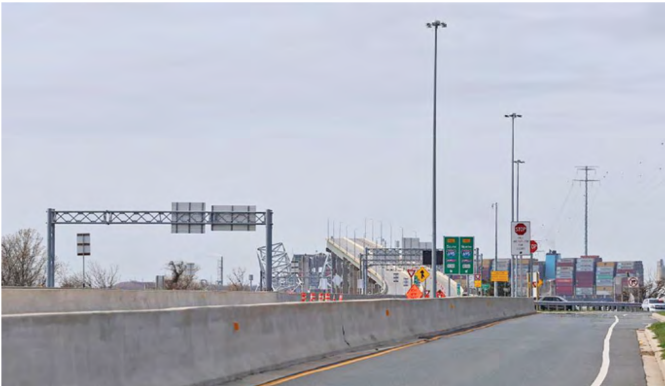
The collapsed Francis Scott Key Bridge in Baltimore, Maryland, US (Xinhua)
