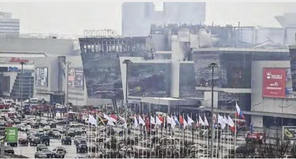
A view of damage at Crocus City Hall concert venue near Moscow, Russia
