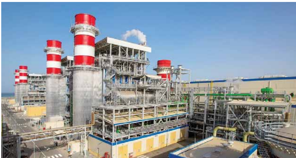
With the exception of Ibri II, all the generators participating in the Oman Electricity during 2023 were conventional gas-powered plants.
