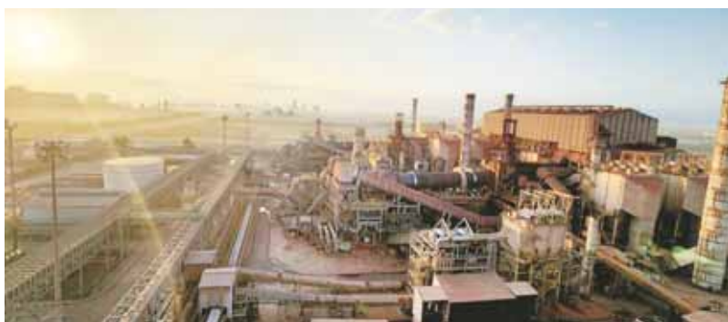
Vale Oman's pelletising complex at Sohar Port.
