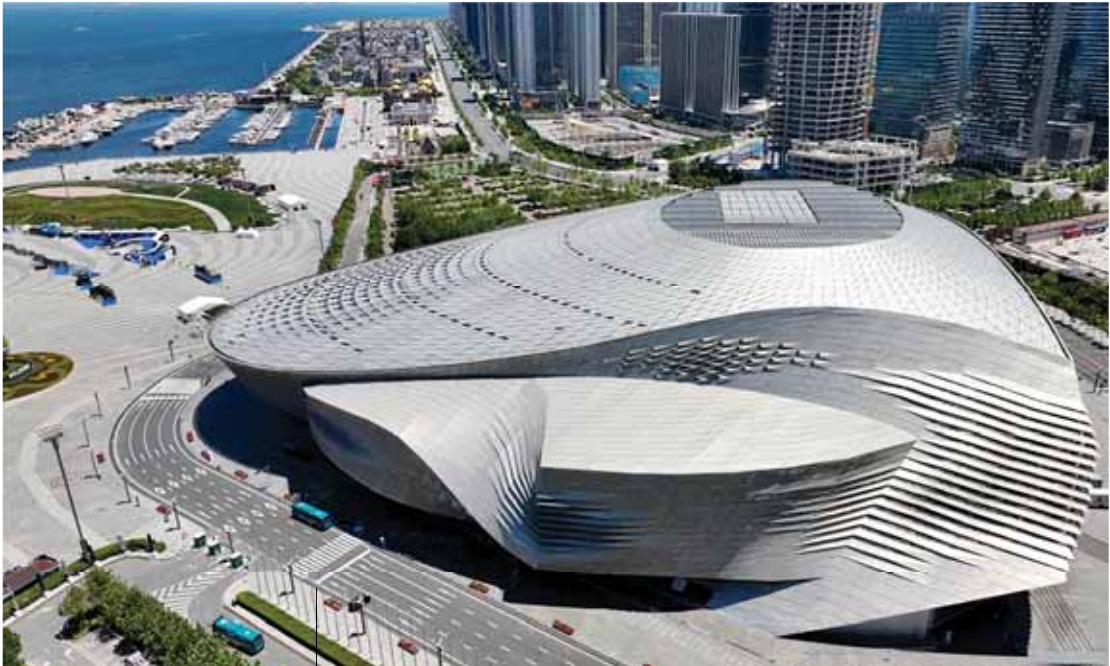
Venue of 2024 Summer Davos An aerial drone picture shows the Dalian International Conference Centre, venue of the 2024 Summer Davos, in Dalian, northeast China's Liaoning Province. Xinhua
