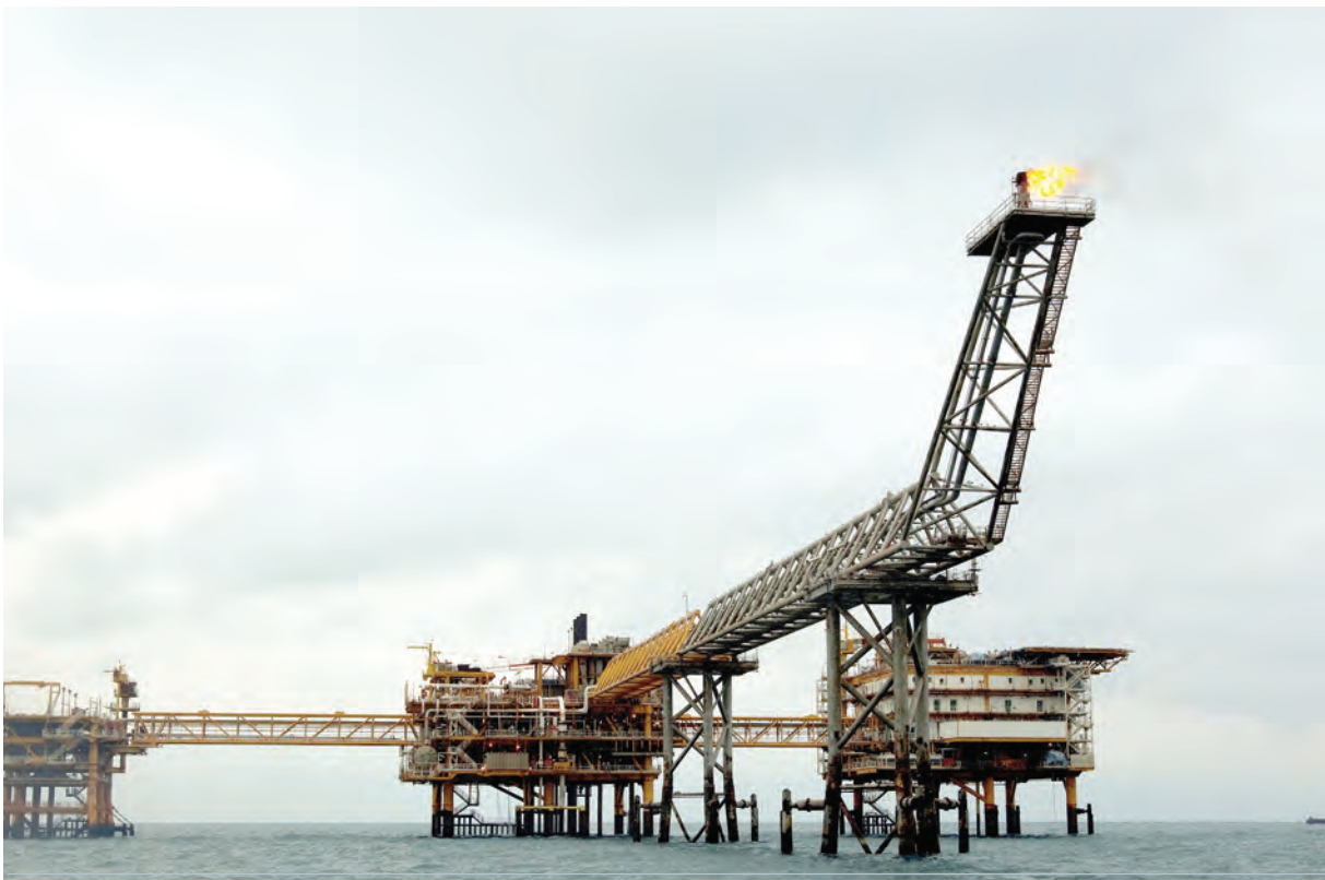
The SPQ1 gas platform is seen on the southern edge of Iran's South Pars gas field in the Gulf. — Reuters
