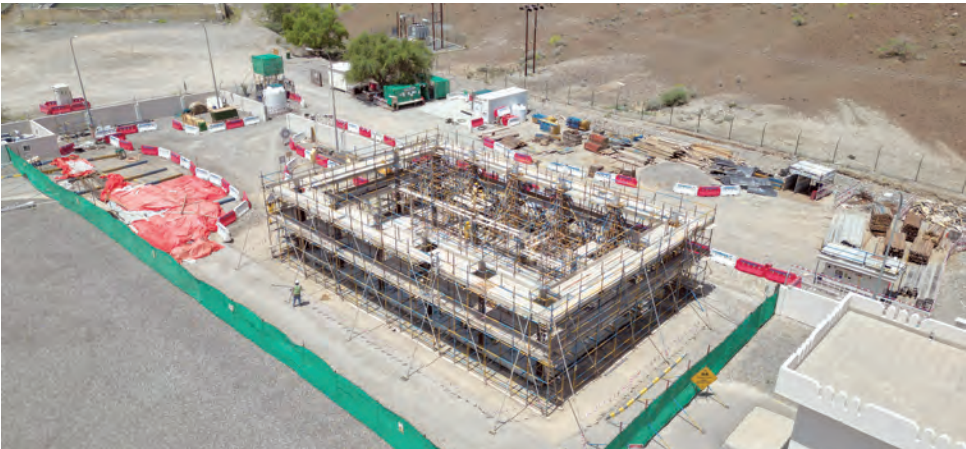
Upon completion, the project will provide more than 840 household connections, benefiting approximately 4,200 residents and improving the reliability and accessibility of water services in the area.
