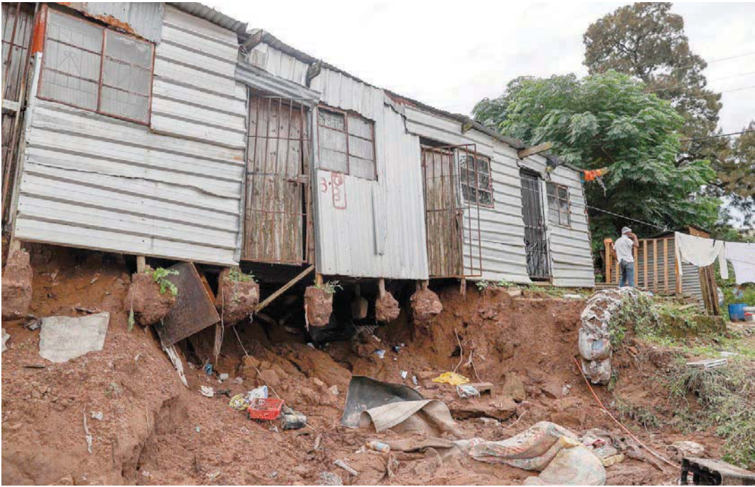
A general view of a damaged structure after a mudslide destroyed the floor near Durban. — AFP
