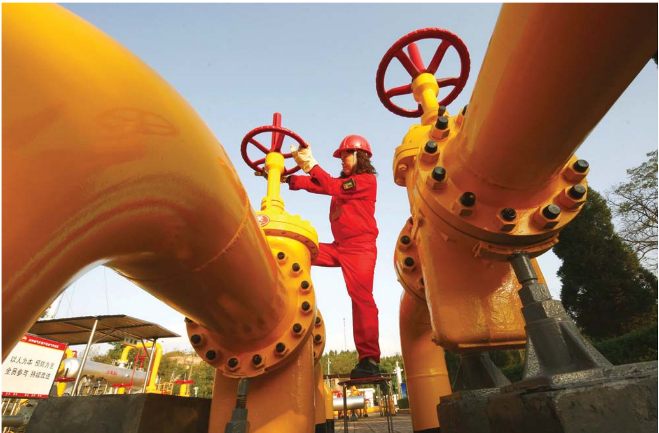
A Chinese worker checks the valve of a gas pipe at a natural gas plant in Suining, in southwest China's Sichuan province. — Reuters
