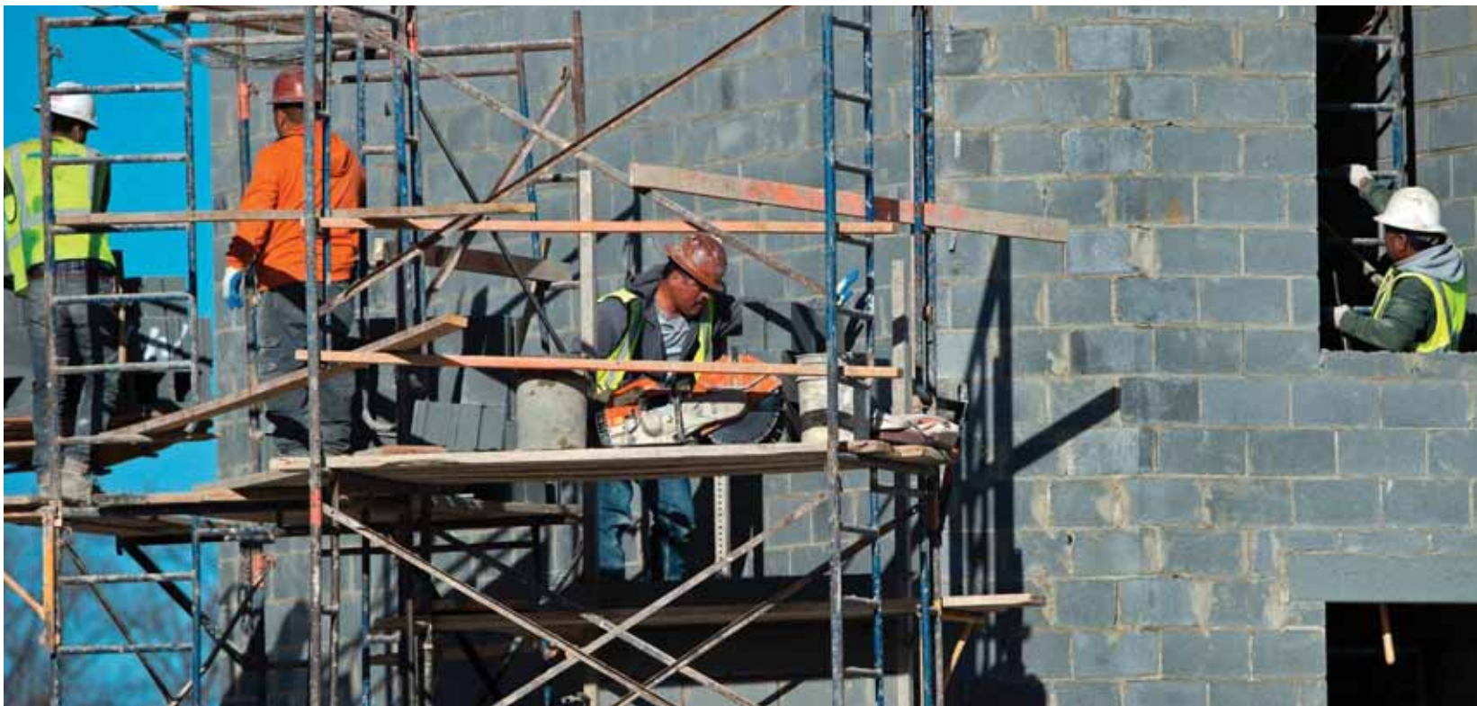
Construction workers are seen as they build an apartment building in Fairfax, Virginia. — AFP
