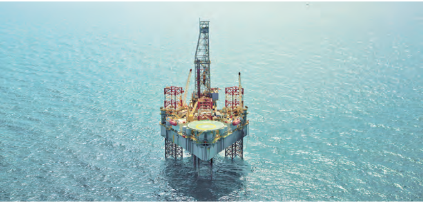
The new flowline became operational in late January 2025, allowing the seamless transfer of produced fluids from the field.
