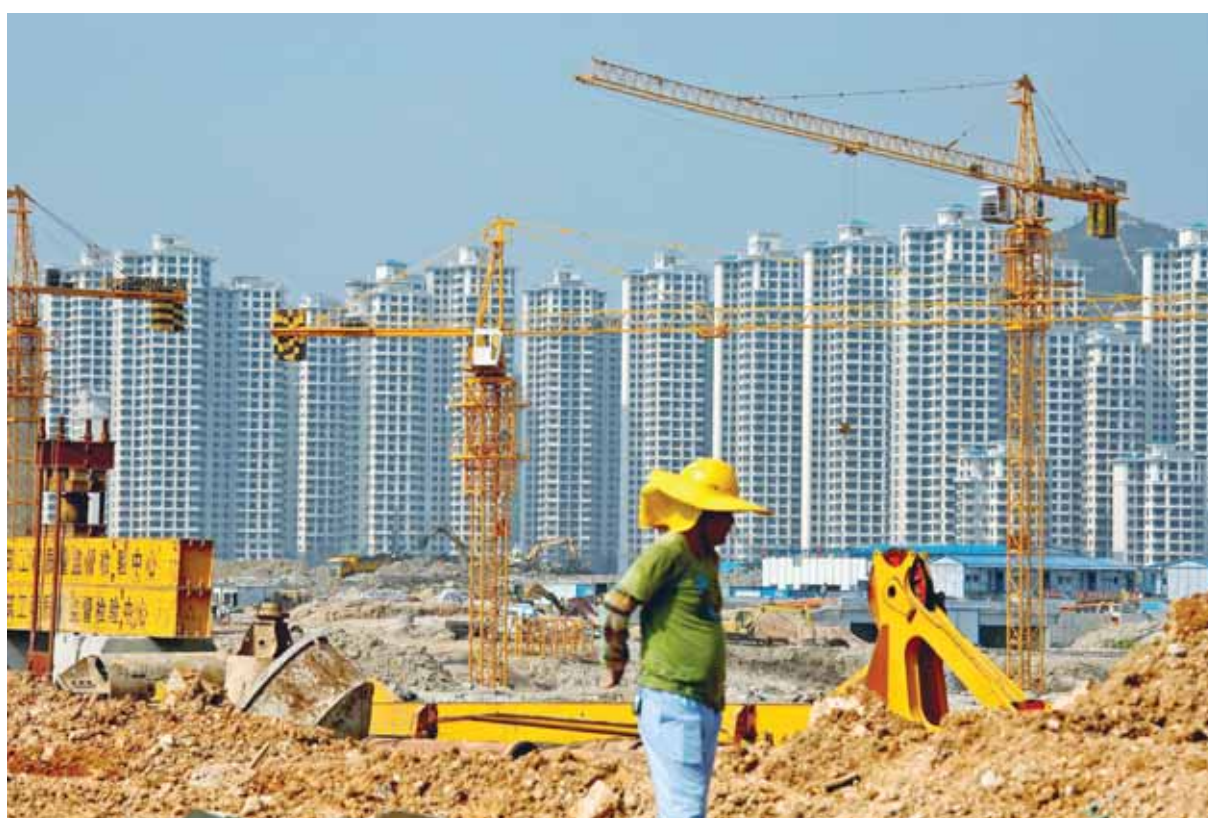
Residential apartments are under construction at Hengqin Island, China. — Reuters
