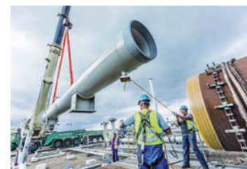
Pipeline parts are installed at Nord Stream 2 receiving station in Lubmin, Germany. — Reuters
