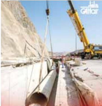
Under the contract, Galfar will construct water distribution networks in the wilayats of Ibri, Yanqul and Dhank in Al Dhahirah Governorate.
