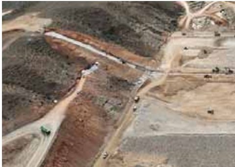
Part of the Wadi Adawnib Dam project under construction in Salalah
