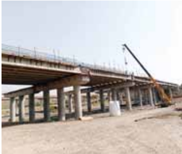
Wadi bridge under construction on the Al Kamil W'al Wafi-Sur stretch.
