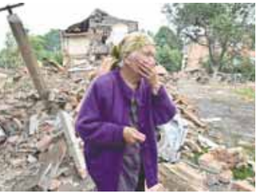
A resident reacts next to a damaged building partially destroyed after a shelling in the city of Chuguiv, east of Kharkiv, on Saturday. – AFP
