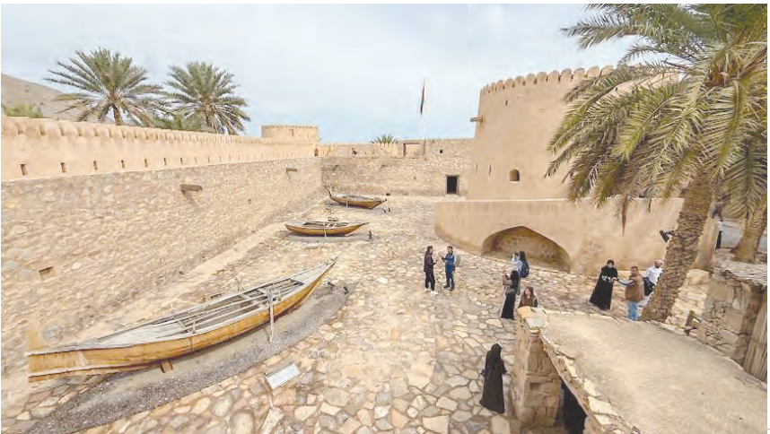
The number of visitors to Khasab fort, which exceeded 6,000 by the end of October 2025 before its closure for restoration and maintenance works, reflects its continued importance as one of the governorate’s prominent historical and tourist landmarks.
