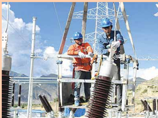
Chinese electricians check and repair electricity grids and power transmission equipment in Yichang city, central China's Hubei province. — Reuters
